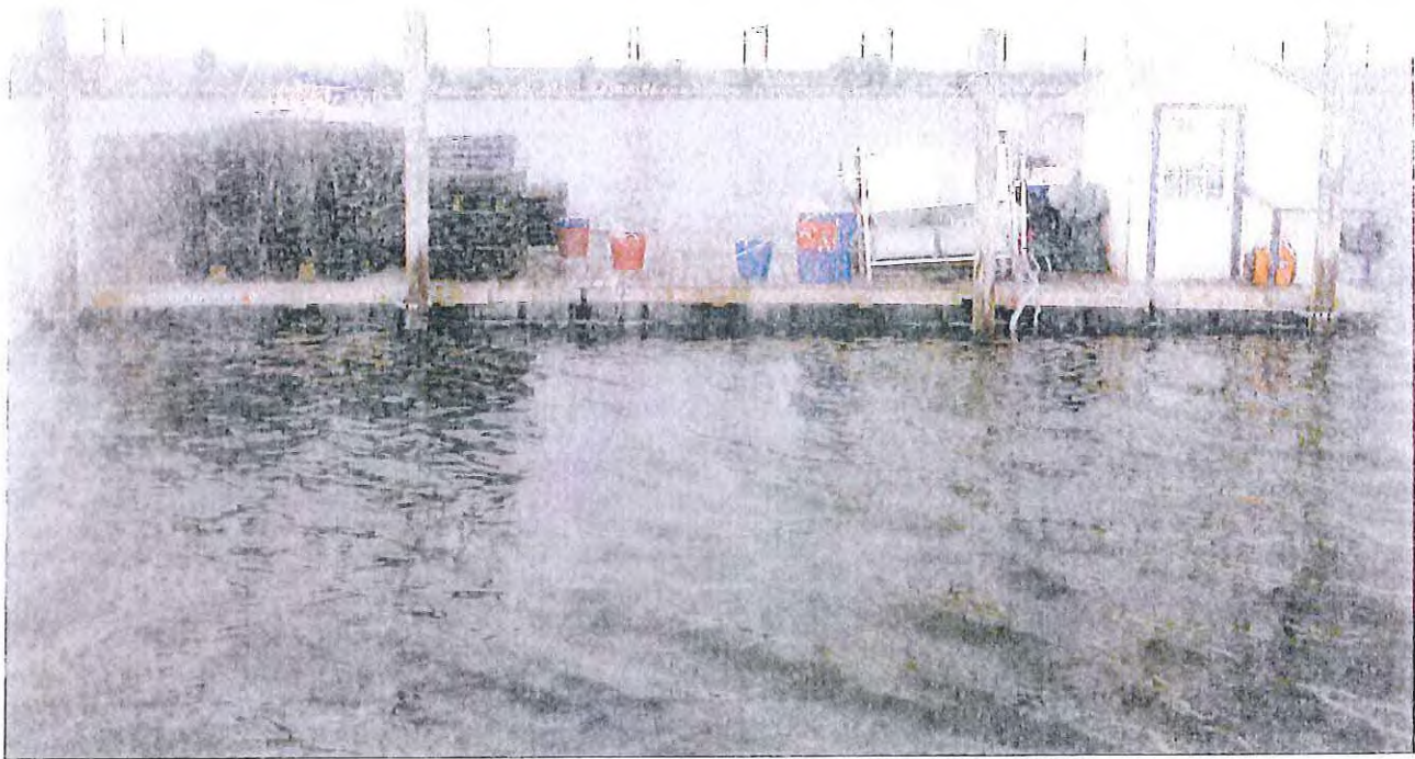
Picture of four existing Pilings and Vessel-looking SSW.
